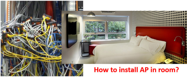
Traditional challenges on laying additional cabling for AP installation
